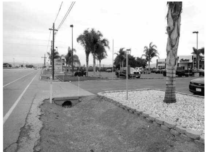
Shallow uncovered stormwater drain by the bus stop
