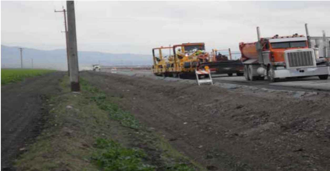
Paving Stage 2 Shoulder
