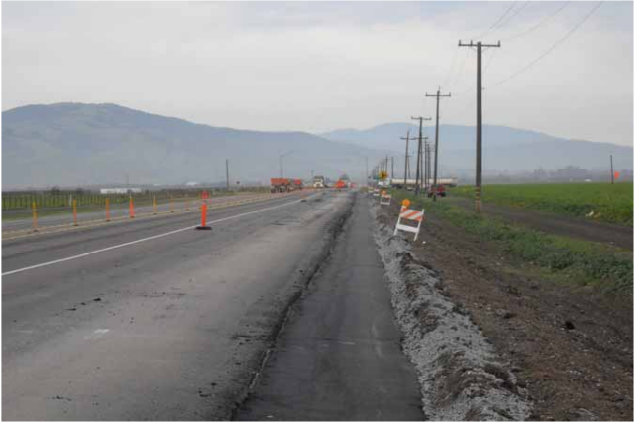
Shoulder Widening on Stage 2
