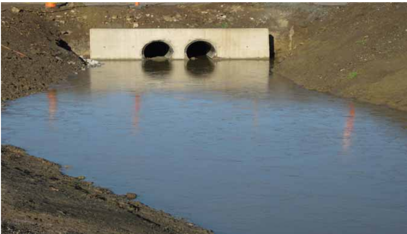
Drainage System at Shore Rd with new Headwall
