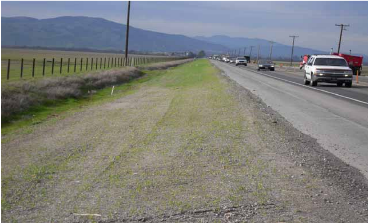
Stage 1 Hydro seeding
