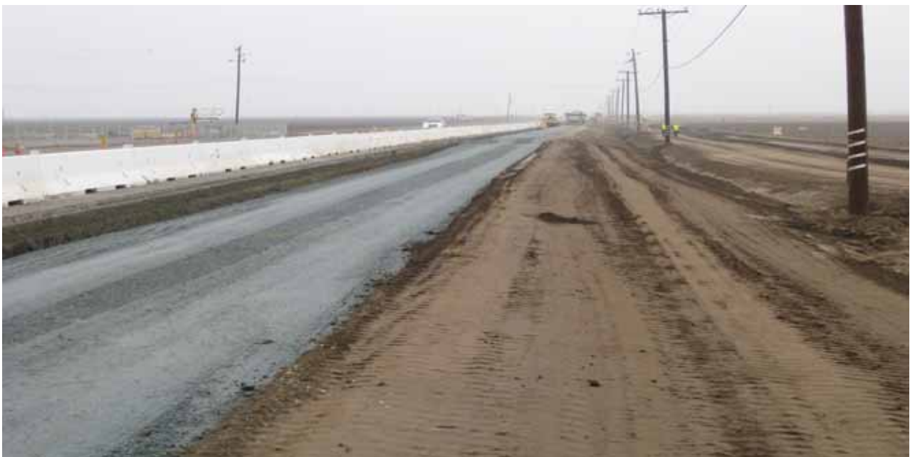
Embankment on Stage 2
