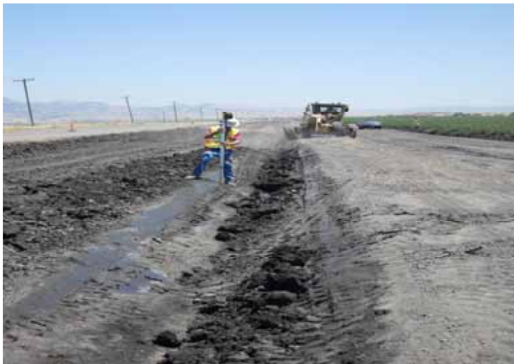
Pavex Checking Grade
