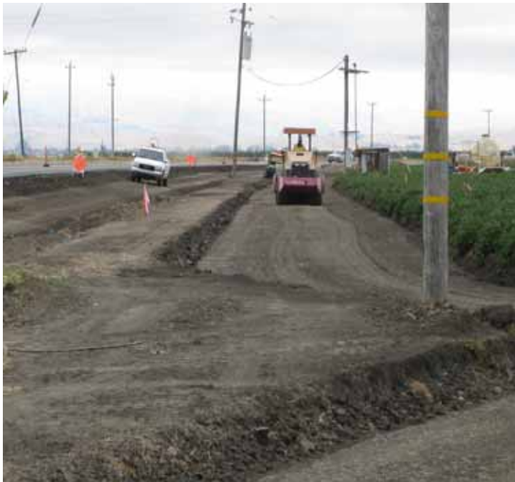
Compaction on Access Road
