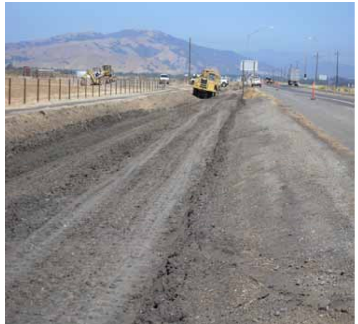
Embankment Area at Shore Road
