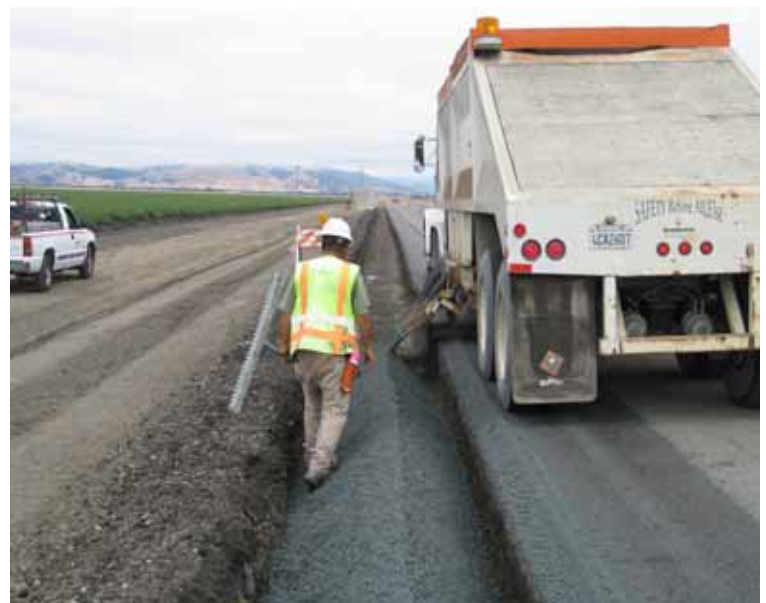
Pavex Placing Base on Shoulder
