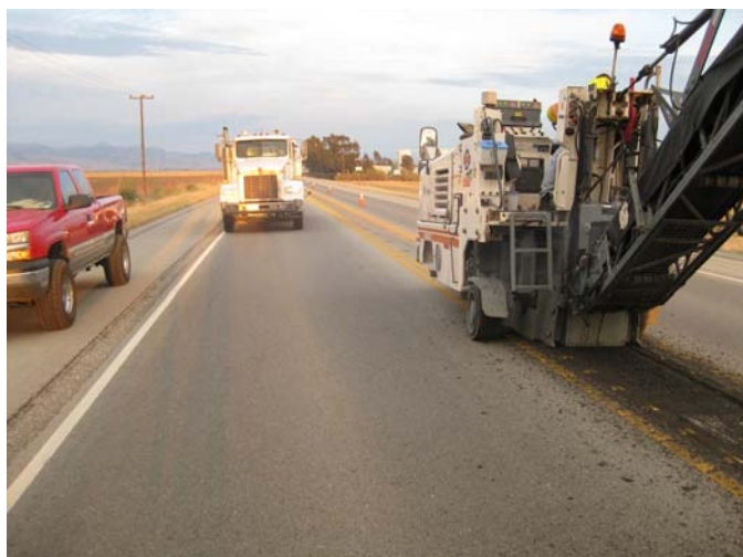
Remove / Re-pave Rumble Strips
