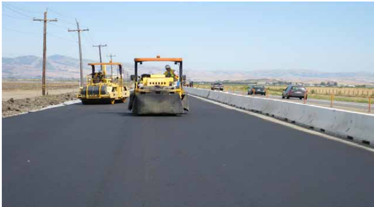
Widening at Shore Rd.
