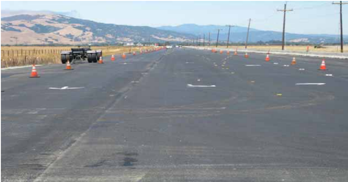
Overlay on Hwy 25 with new Turn Lane on to Shore Rd
