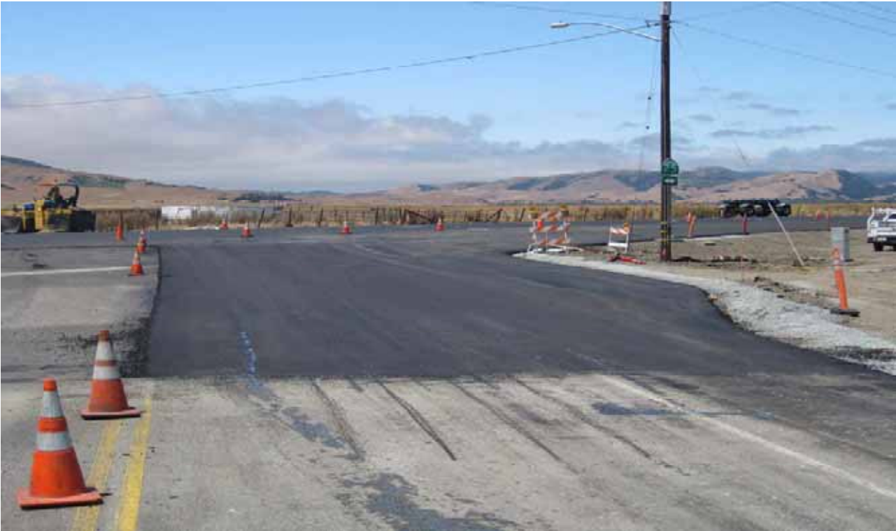
Overlay with Turn Lane to Hwy 25 Northbound
