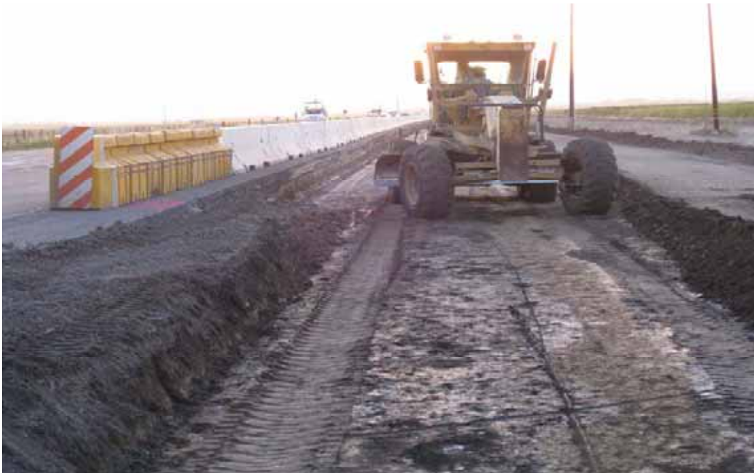
Widening At Shore Rd. Stage 2
