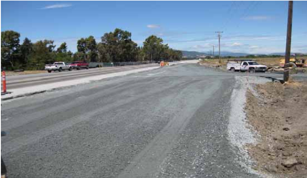
Widening at Tri Cal
