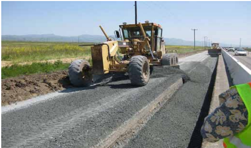
Stage 2 Traveled way section placement of Class 2 Base
